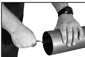
Figure 3: Deburr inside diameter deburring tool
