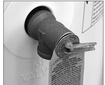
Figure 24 - Temperature and Pressure Relief Valve
