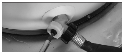
Figure 39 - Draining the water heater.
