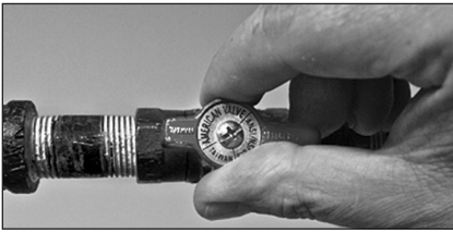
Figure 49 - Gas valve in "on" position.
