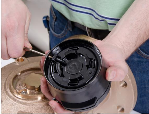
Figure 8 – Removing the Seal Pin
