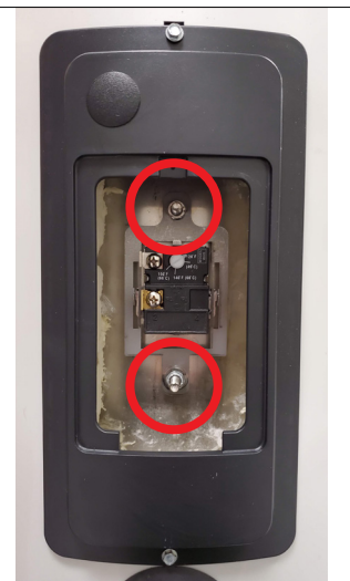
Figure 18 - Nuts Securing the Thermostat
