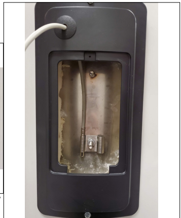
Figure 22 - Sensor Clip on the Lower Stud
