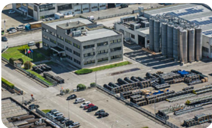
Production Facility - Castel Guelfo di Bologna (BO)
