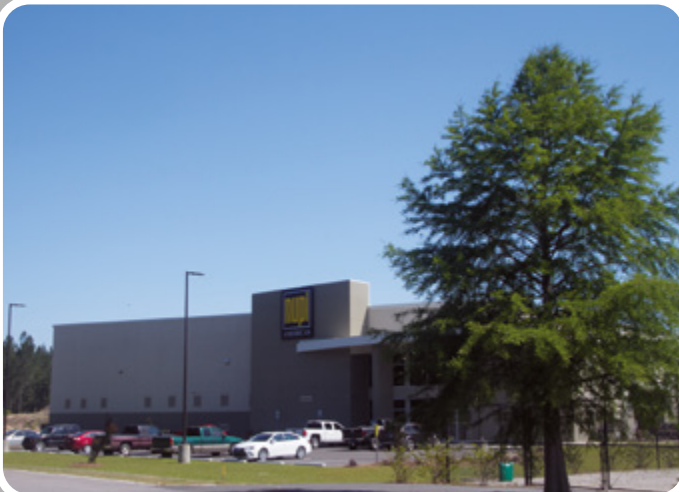
Production, Operations & Administration Center - NUPI AMERICAS INC. - Early Branch (SC)
