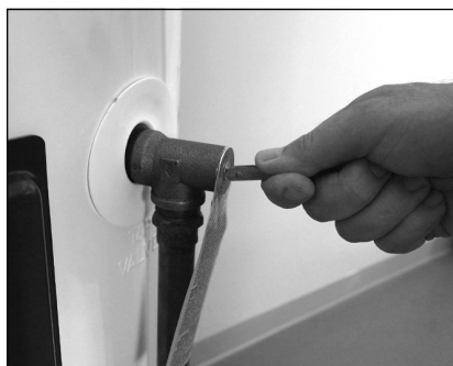
Figure 38 - T&P Relief Valve
