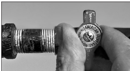
Figure 2: Turn the gas control valve off.
