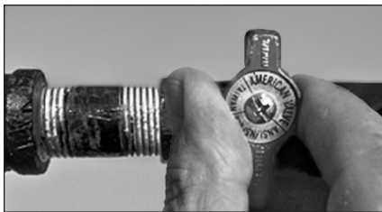
Figure 2: Turn the gas control valve off.
