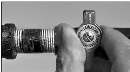
Figure 2: Turn the gas control valve off.
