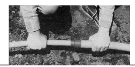
**3.** Slide washer, retainer, gasket, and lock ring over pipe. Refer to photograph for correct assembly.
