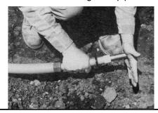
**5.** Insert pipe with components into body. Slide riser casing forward and thread nut onto body.
