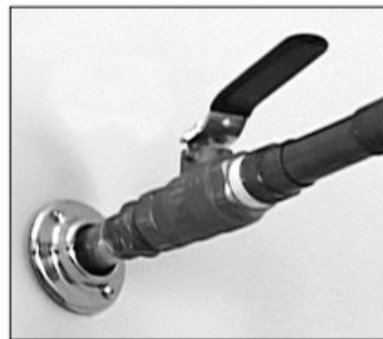
Figure 20 - Fully open the cold water supply valve (full-flow ball valve pictured above).
