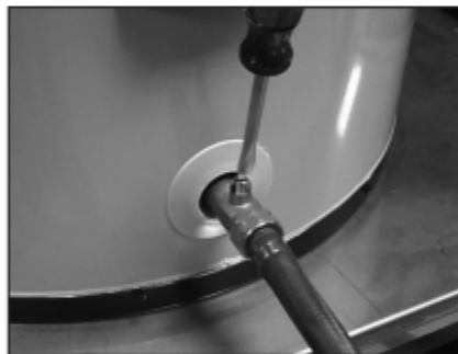
Figure 11 - Draining the old water heater.
