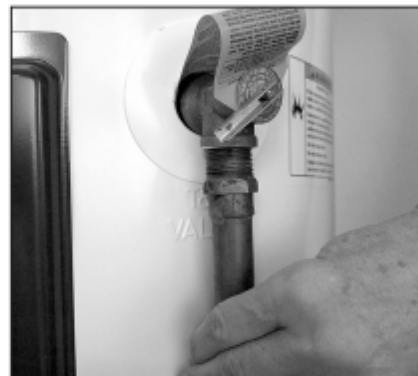
Figure 15 - The T&P Relief Valve discharge pipe must be installed properly and piped to an adequate drain.
