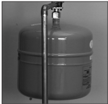
Figure 6 - A Thermal Expansion Tank helps protect the home's plumbing system from pressure spikes.
