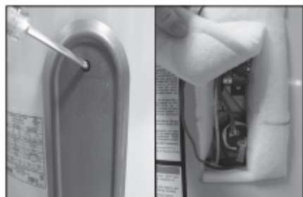
Figure 48 - Element Access Panel/ECO Compartment.
