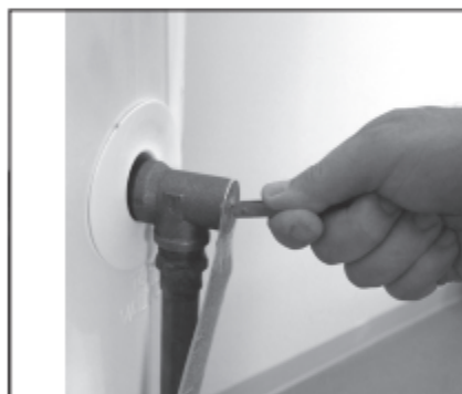
Figure 49 - T&P Relief Valve.
