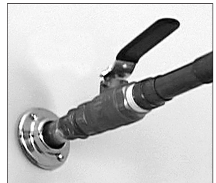
Figure 21 - Fully open the cold water supply valve (full-flow ball valve pictured above).
