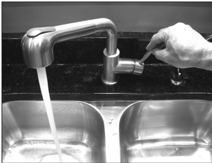
Figure 10 - Let the hot water run until it is cool.
