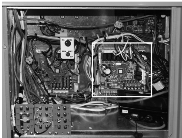
Figure 11. Precedent™ B Cabinet - RTRM board
