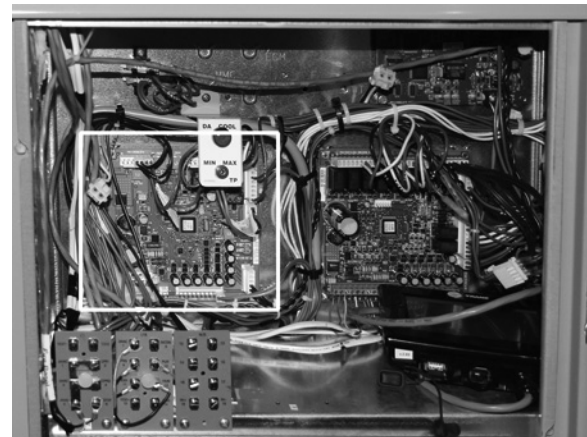
Figure 13. Precedent™ E Cabinet - RTOM board
