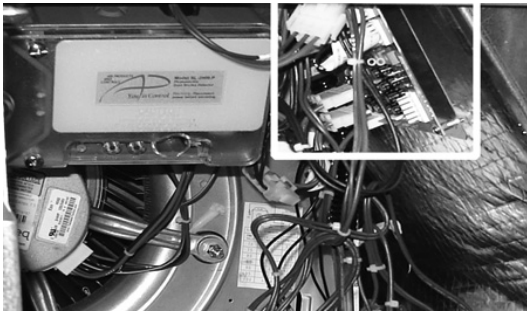
Figure 15. Precedent™ B Cabinet - RTOM board
