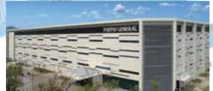
Fujitsu General Air Conditioning R&D (Thailand) Co., Ltd. (Thailand)
