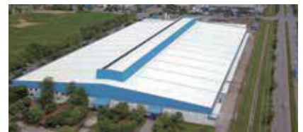
Fujitsu General (Thailand) Co., Ltd. (Thailand) FACTORY-2
