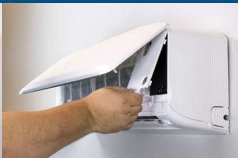
Remove electrical access panels (2)
