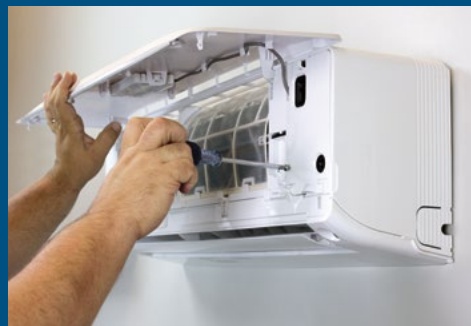
Back out electrical panel screws
